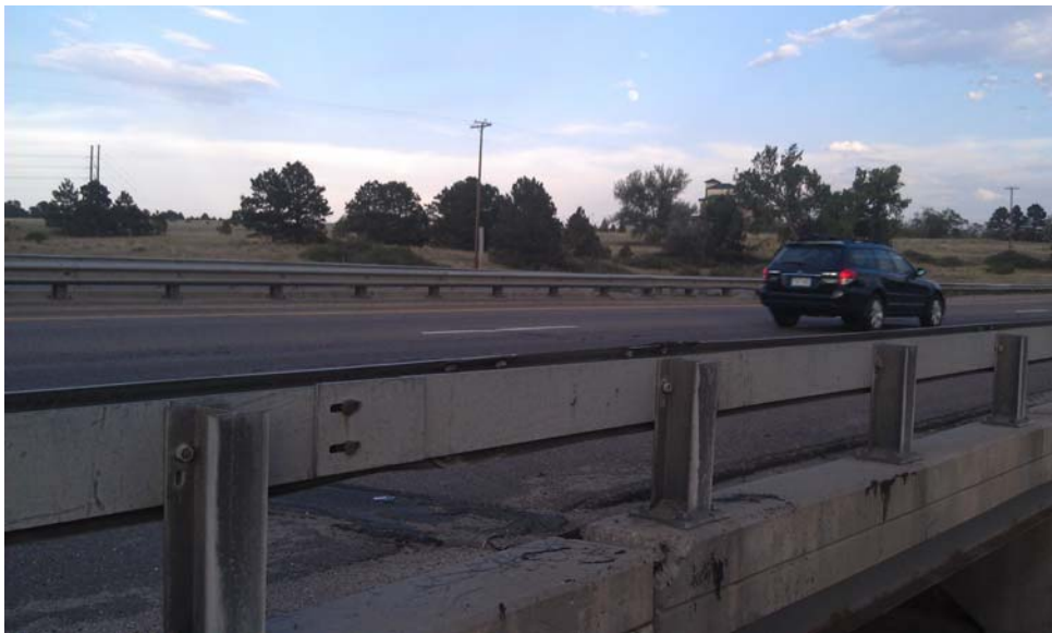
Photo 1 – View of Bridge Structure ID: H-17-J.
